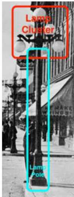
The 1910 design showing the two components of the original street light consisting of the lamp pole (later installed at in Massey and Victory Heights) and original cluster lamp top (replaced by single globes in 1926). Detail from New Westminster Archives photo 2397.
